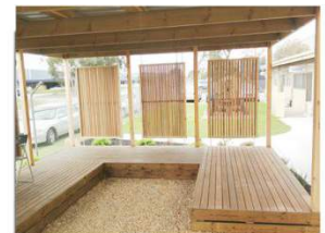
Products are finished to profile and lengths required for the job
